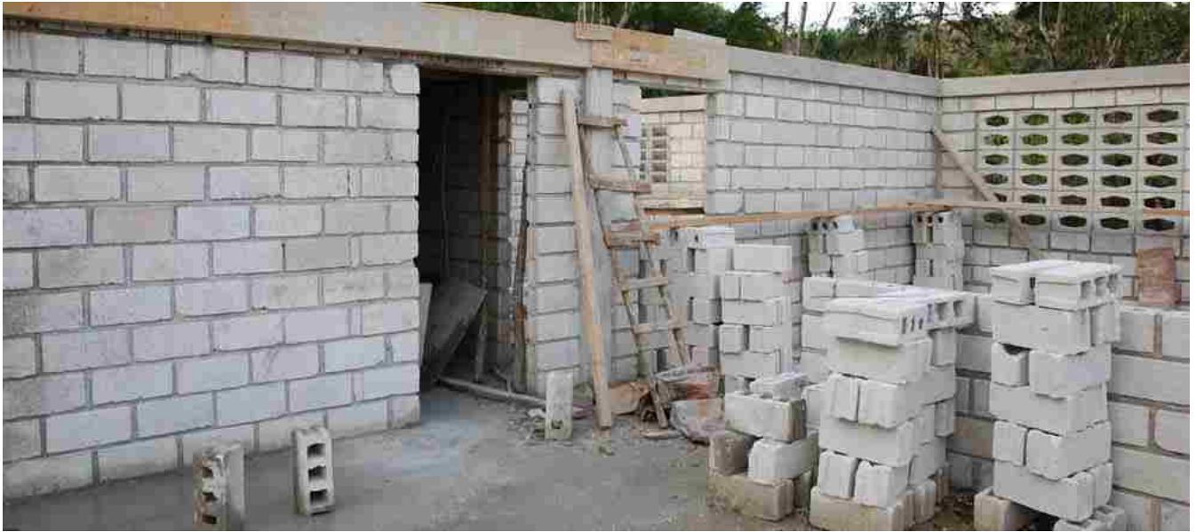
Fig. 4.6: Concrete Block Construction
