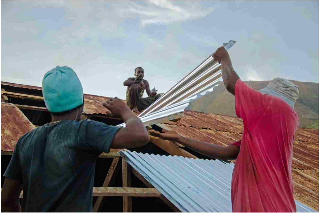
Fig. 4.9: Open Society Foundations Corrugated Metal Roof
